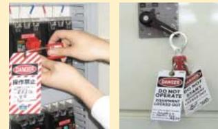
Lock-out and tag-out Example when multiple workers are at work
