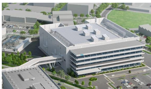
Koshi-city, Kumamoto Prefecture Completion scheduled for summer 2025
