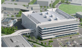
Koshi-city, Kumamoto Prefecture Completion scheduled for summer 2025
