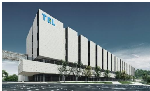
Kurokawa-gun, Miyagi Prefecture Completion scheduled for summer 2027
