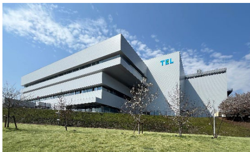
Kurokawa-gun, Miyagi Prefecture Completed in April 2025
