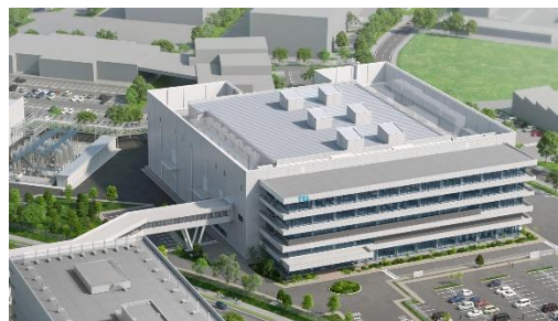
Koshi-city, Kumamoto Prefecture Completion scheduled for summer 2025
