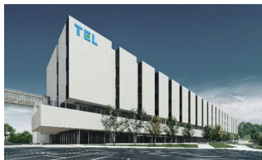
Kurokawa-gun, Miyagi Prefecture Completion scheduled for summer 2027
