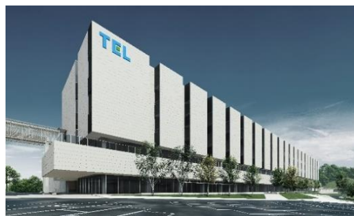
Kurokawa-gun, Miyagi Prefecture Completion scheduled for summer 2027
