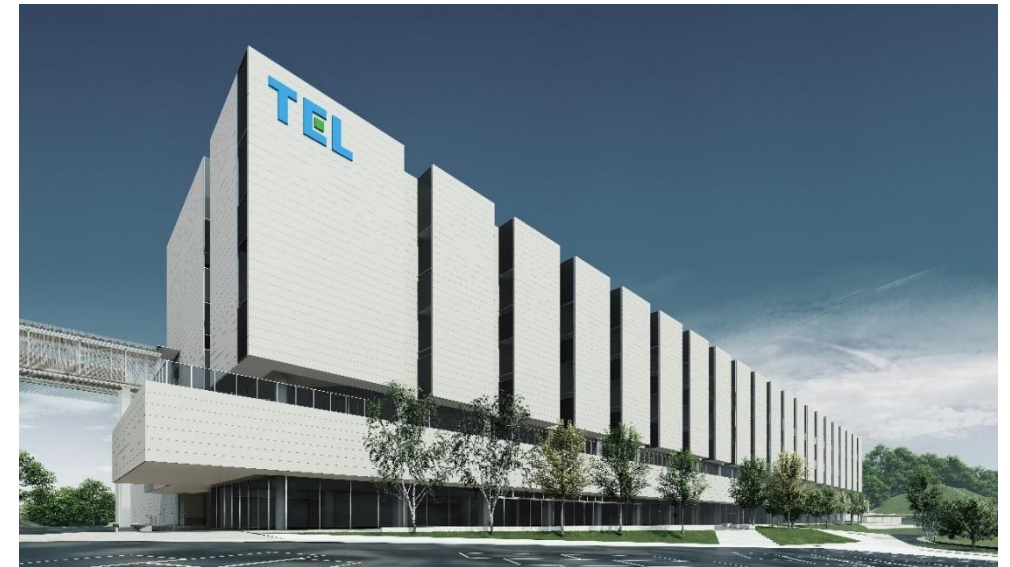
Miyagi innovative Production Center (Completion scheduled for summer 2027)
