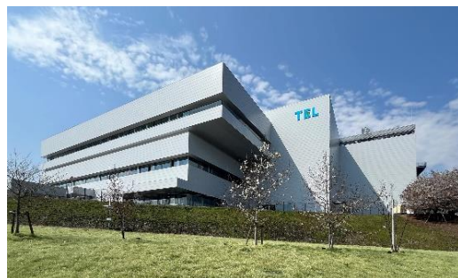
Kurokawa-gun, Miyagi Prefecture Completed in April 2025
