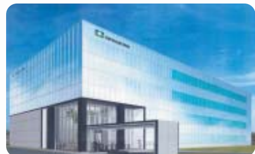
Tokyo Electron (Shanghai) Limited New Headquarter Building
