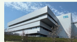
Development Building No. 3, Tokyo Electron Miyagi
