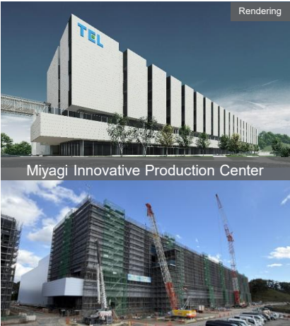
Miyagi Innovative Production Center Taiwa-cho, Kurokawa-gun, Miyagi Prefecture Completion scheduled for summer 2027
