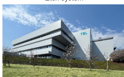
Kurokawa-gun, Miyagi Prefecture Completed in April 2025
