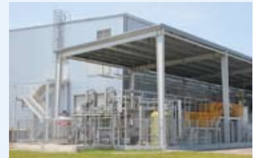
Synthetic wastewater treatment facility
