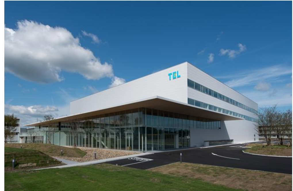
Tokyo Electron Miyagi's Miyagi Technology Innovation Center
