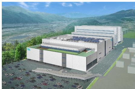
Nirasaki City, Yamanashi Prefecture: approx. ¥13.0B construction cost (Scheduled to begin operation in August 2020)
