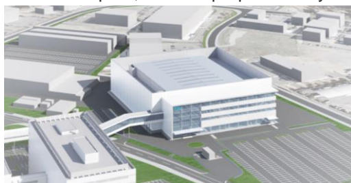
Koshi-city, Kumamoto Prefecture: approx. ¥30.0B construction cost (Completion scheduled for fall 2024)
