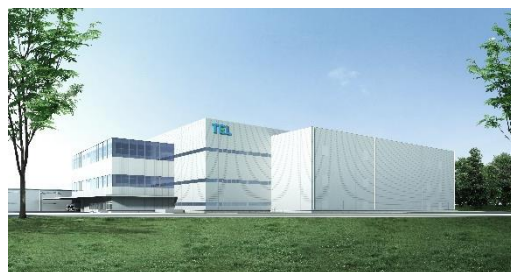
Kurokawa-gun, Miyagi Prefecture: approx. ¥47.0B construction cost (Completion scheduled for spring 2025)
