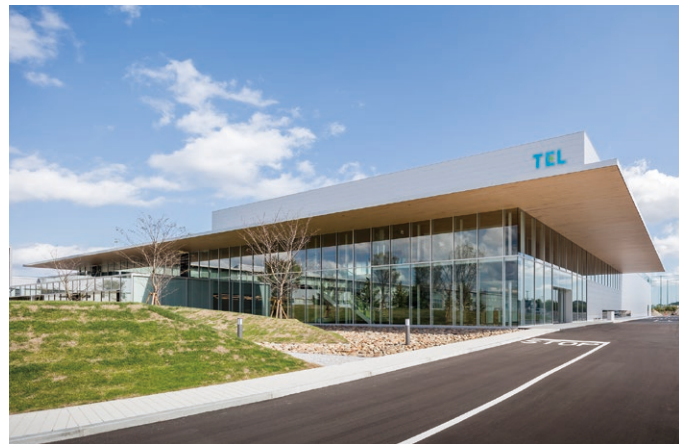
Head Office: Miyagi Technology Innovation Center
