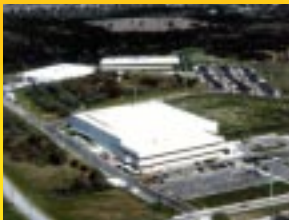
Tokyo Electron Texas, Inc., shown with Tokyo Electron America, Inc.'s head office and parts and training center in the background, produces advanced CLEAN TRACK coater/developers.
