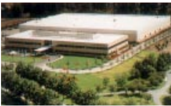
Since building Tokyo Electron Oregon, our first U.S. manufacturing facility, we have added others to ensure timely response to customer demands.
