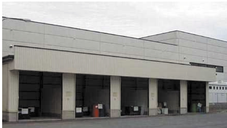
Waste storage facility (Tohoku Plant)
